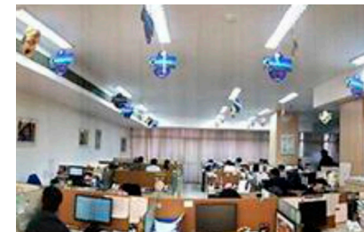
An office at Nikon India Private Limited, where LED lights are now used for almost all the lighting
