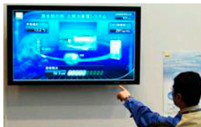
Monitor showing the amount of power generated in real time at the Kumagaya Plant
