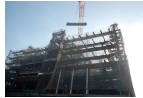
Ceremony of putting up the ridge beam (September 2023)
